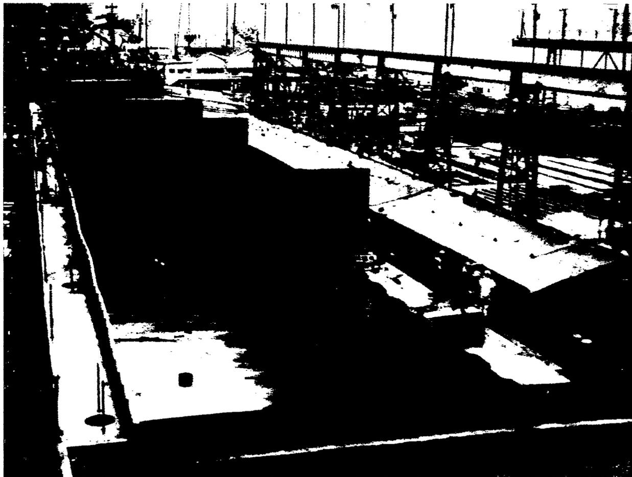
**Figure 48—Barge Construction Showing a Side Shell Unit (at right) in Horizontal Position Ready to be Erected Into Final Vertical Position**
